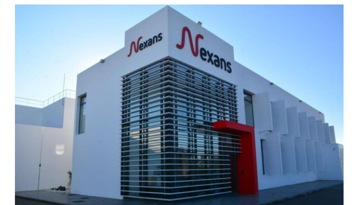
Jan. 19 - Nexans inaugurates a new plant in Morocco for the production of fiber optic cable accessories
